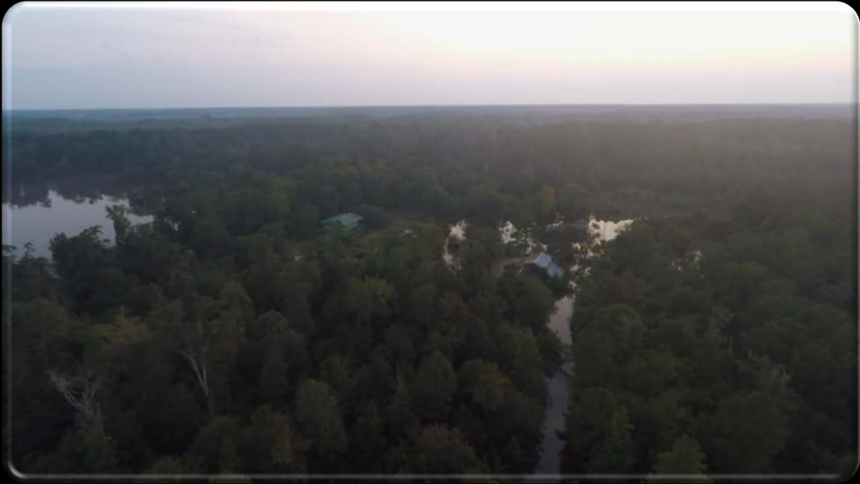
Big Thicket National Monument, Texas Hurricane Harvey damage assessment
