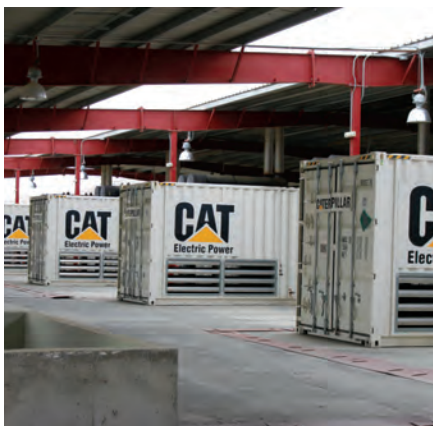
Diesel generators are used to provide electricity until NEPS and SEPS can be expanded and connected. (SIGAR photo by Steven Mocsary)
